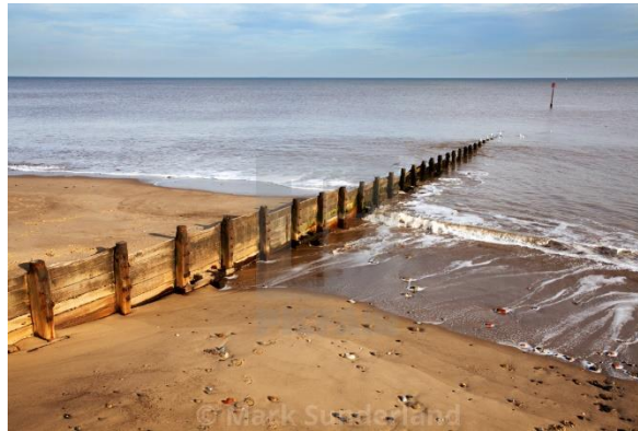
Wooden groynes on Hornsea beach
