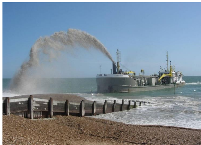
Beach nourishment going on at Hayling Island
