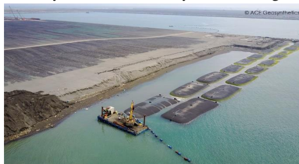
Geotextile tube at Harbour, Kaohsiung, Taiwan
