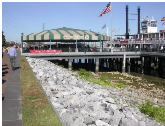
Revetment near the ferry dock at Jean Lafitte National Historical Park and Preserve, Louisiana. (National Park Service)
