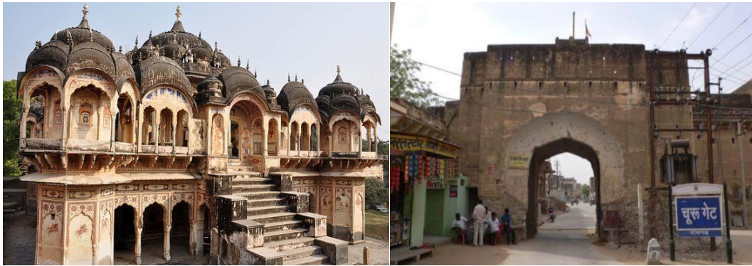
Figure 12. Major urban elements (i.e. Garh, Haveli, Chattri, gateway to town) in settlement of Ramgarh.
