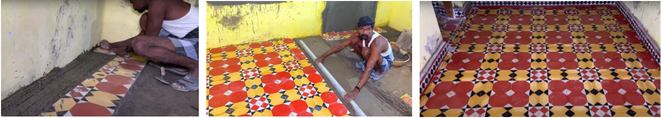
Fig.2.1.8 Tile laying process
