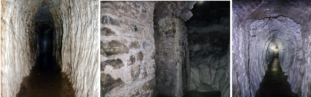
Figure 3, 4 & 5: Underground water channel of Kundi Bhandara, Burhanpur, Madhya Pradesh
