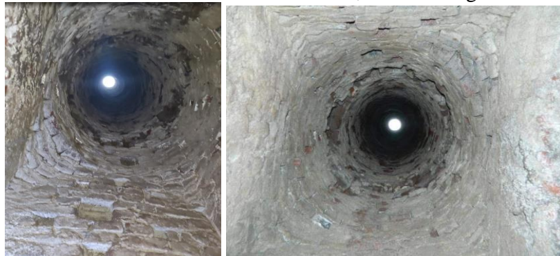
Figure 9 & 10 : Internal view of Air Shafts- Kundis, from underground water channel
