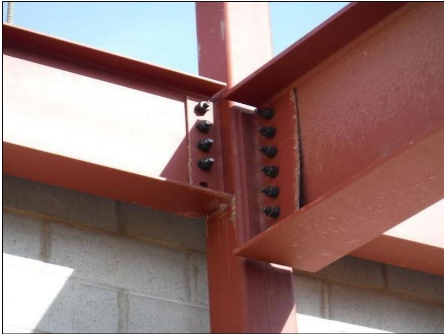
Fig 1.1 Bolted Framed Connections
