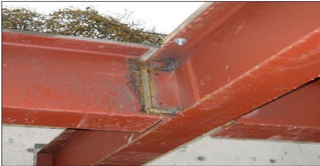
Fig 1.3 Welded Framed Connections
