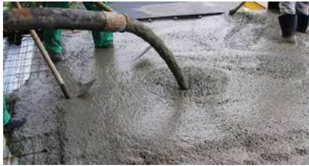
Fig4: Self compacting concrete
