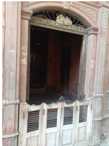
Fig.12a,b & c The external wall surfaces are carved and textured so that the area should increase hence the heat will be distributed (Source: Author)
