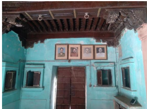
Fig.9 Wooden ceiling for heat insulation (Source: Author)
