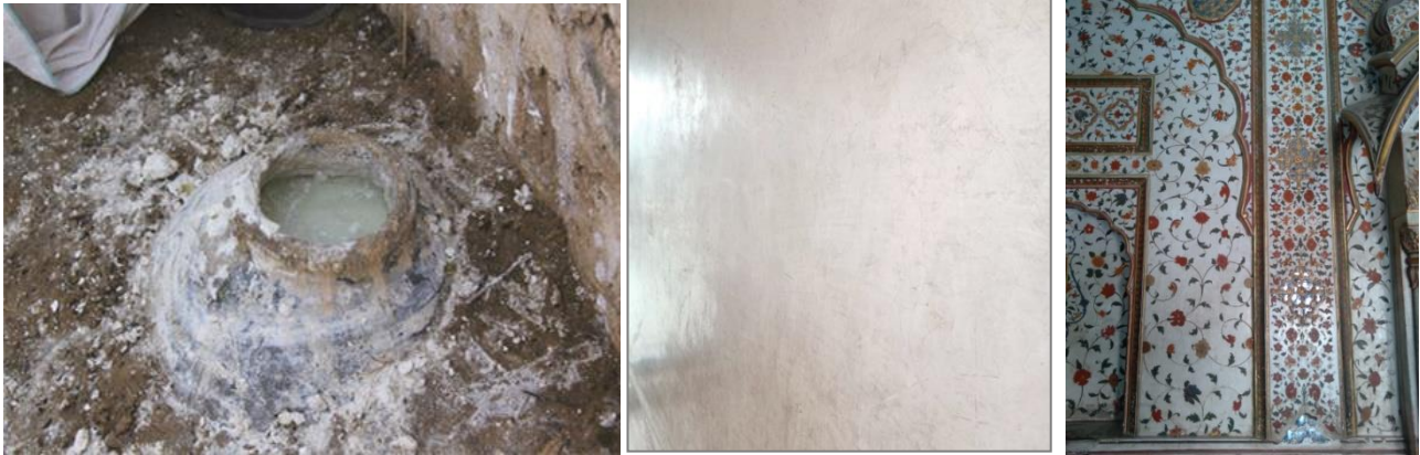
Fig.7a,b,c Araish a Traditional Lime Plastering Process, Finish & application on wall (Source:12a IGNCA. http://asi.nic.in/asi_exca_imp_rajasthan.asp , b&c Author)
