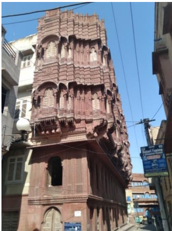
Fig.11a,b & c Jharokhas with jaalis for natural light , ventilation and privacy. Screens lower the air temperature, thus delivering a relatively cooler indoor environment (Source: a&b Author, c- https://cpwd.gov.in/Publication/IGDBooklet )
