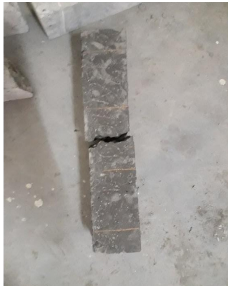
Fig.6.9: Crack in beam specimen
