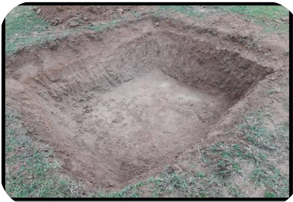
typical 30x40 model pit before harvesting water
