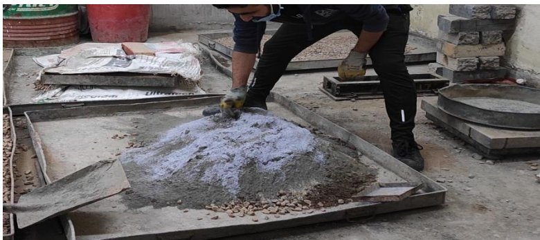
Figure 3. Mixing of concrete.
