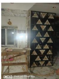
Now these triangle pieces are finished with 3 different types of laminates with the help of adhesive material.
