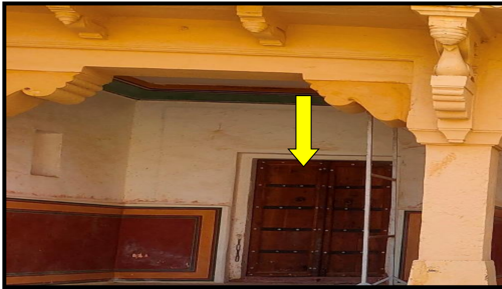
Inner –Hall Wooden Gate
