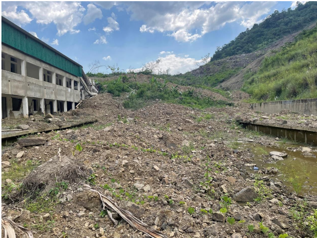
Fig. 8: Tupul landslide (30 th June 2022) Damaged Railway Station and platform
