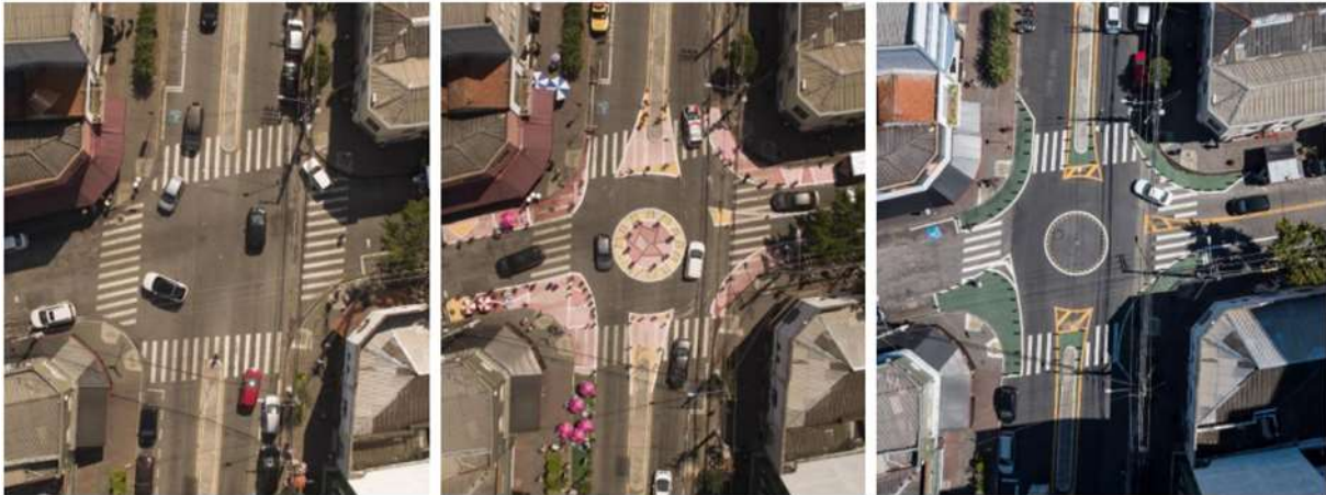
Figure 5: Before, Temporary implementation 2017, Permanent implementation 2018
