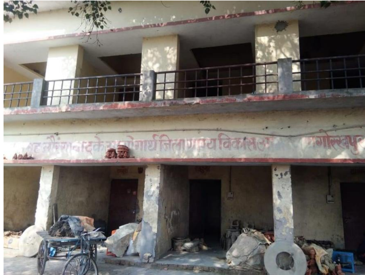
Fig.3. Storage houses in Aurangabad village
