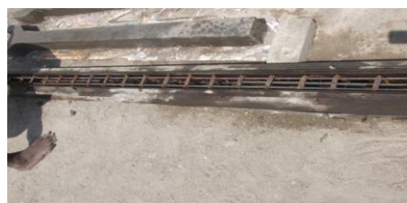
FIGURE 1.4 CASTING OF BEAMS
