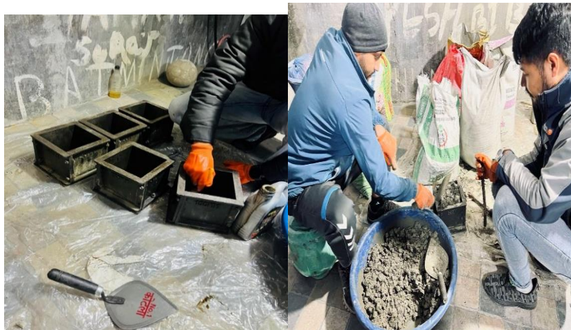
Figure 1: Pictures showing Process from Cube Mold Preparation to Curing
