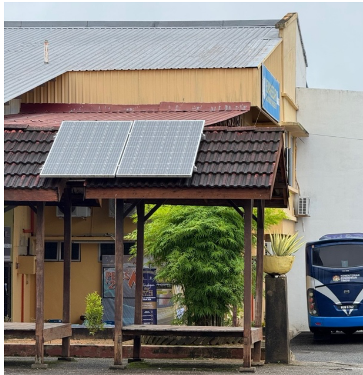
Figure 2: Solar Panel Rooftop Installation at Chenderoh Community College
