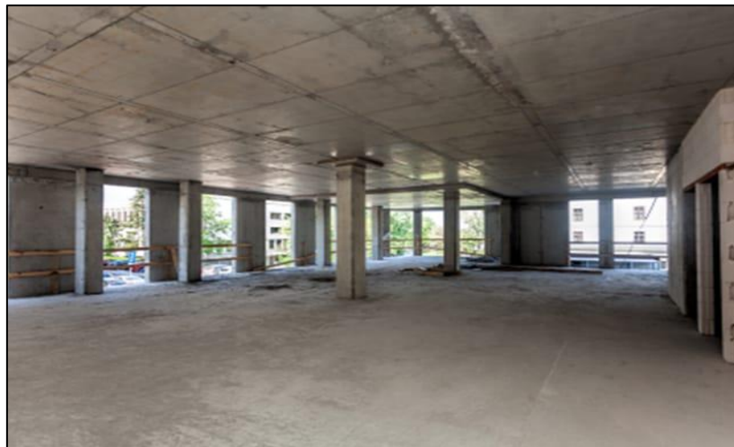
FIG.No.1: TYPICAL FLAT SLAB CONSTRUCTION
