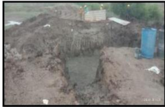
Fig. 04. PCC (plain cement concrete) done on the excavated area for the base.
