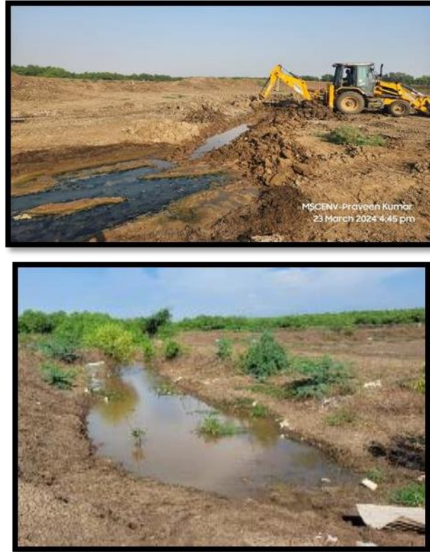
Fig.02. Snap of water overflow from soak pit of traditional septic
