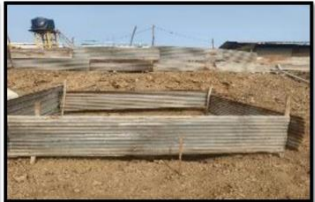
Fig 06. Below Soak pit area made and barricaded using GI sheet to prevent any wild animal entering.
