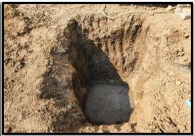
Fig 02. PCC done in the pit for the base, on which bio-digester tank will be placed
