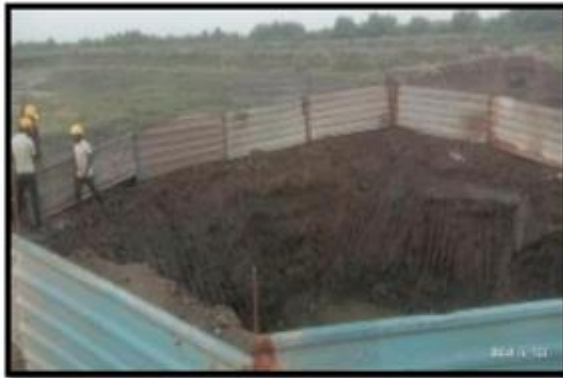
Fig. 03. Excavated area being hard barricaded to prevent personnel, heavy machinery, or wild animals from approaching the pit.
