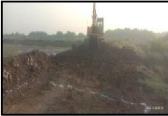
Fig. 01. Layout marking with white lime powder for excavation of the traditional septic tank.
