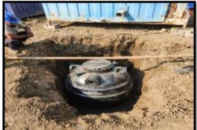
Fig 04. Bio Digester tank was adjusted and sand filling started beside the tank for the support & as per manufacturer guidance.
