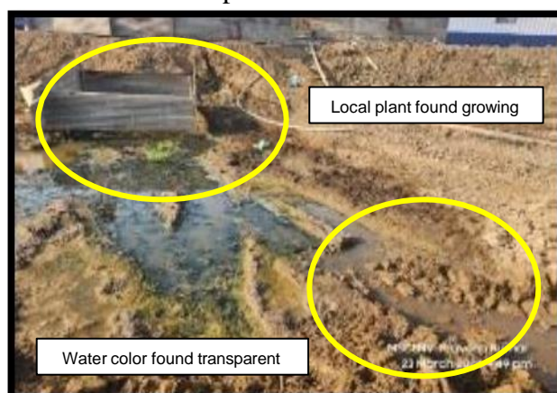
Fig.01. Snap of water overflow from soak pit of Bio digester septic tank
