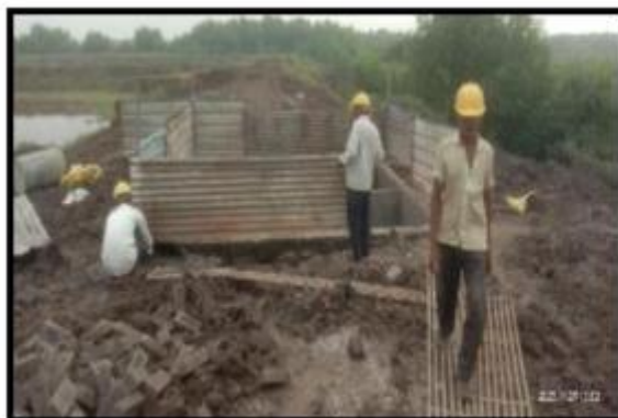
Fig. 05. Partition walls in the septic tank are constructed using masonry work.
