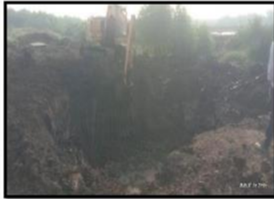
Fig. 02. Excavation for the traditional septic tank using an excavator at the marked location.
