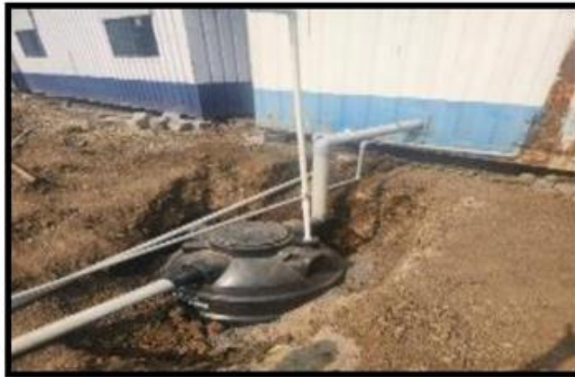
Fig 05. Complete connection Setup of bio digester was done and taken in operational use
