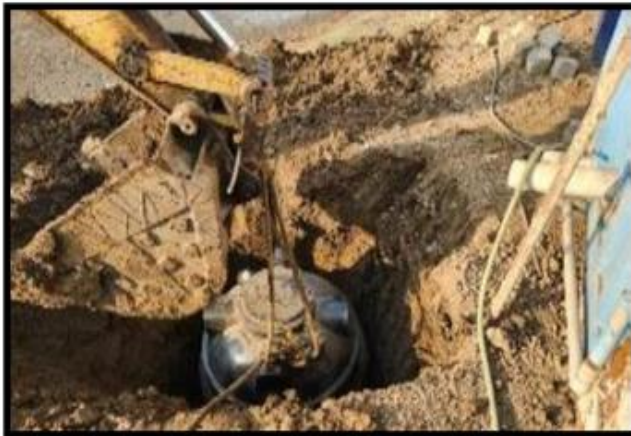
Fig 03. Bio Digester tank was placed in the pit using backhoe bucket
