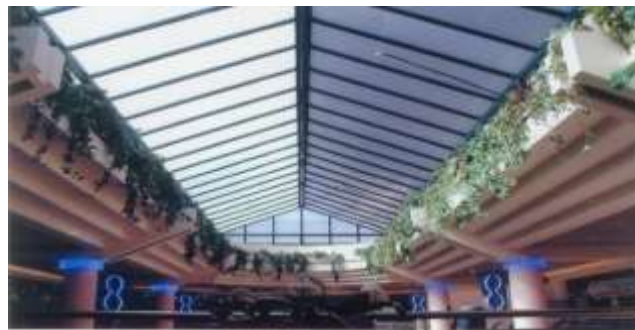
Figure 10 Image Shows Roof Glazed Skylight
