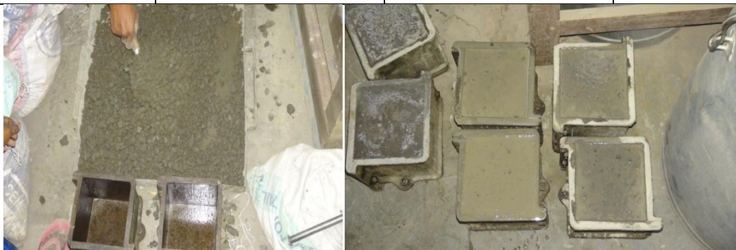
a) Mixing of Concrete Ingredients
