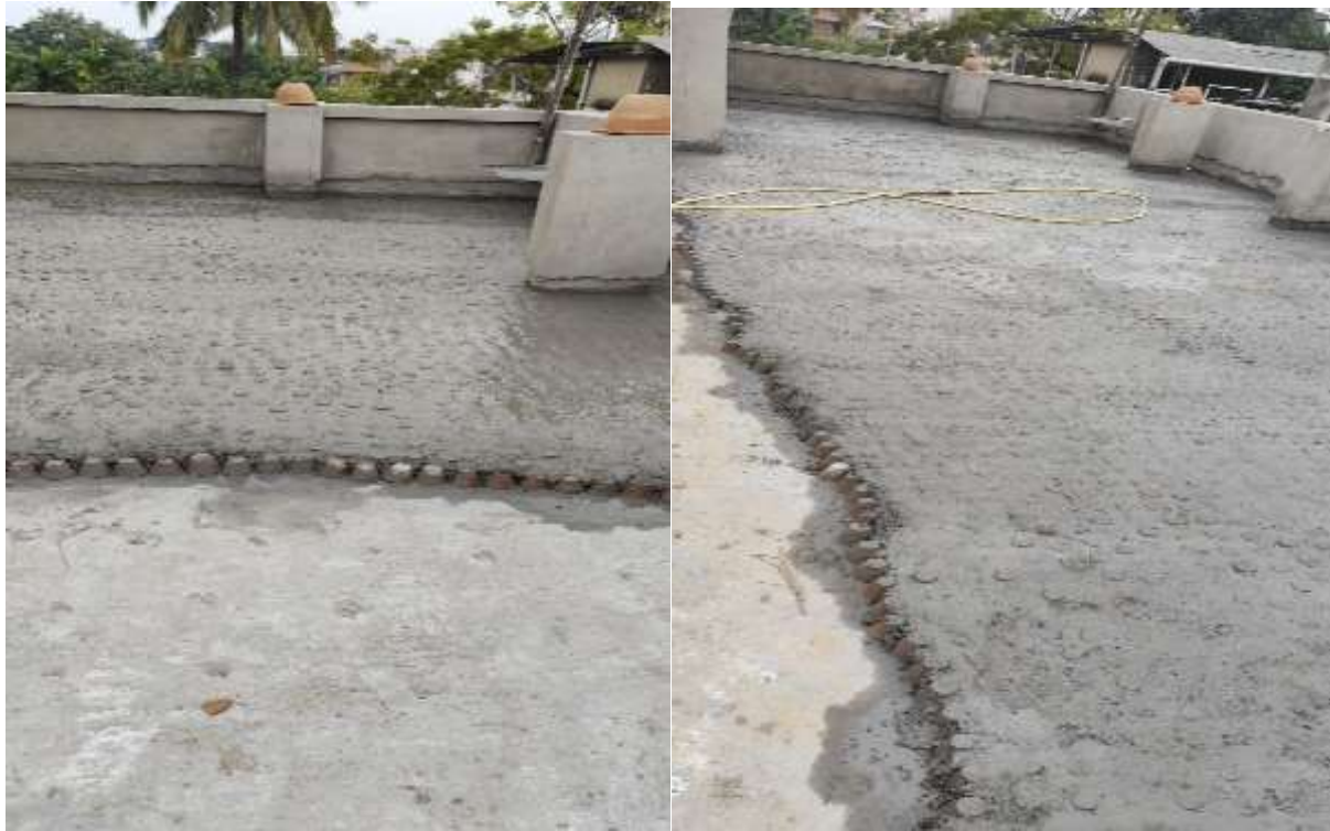
Figure-3.8 Water proofing and heat insulating treatment over roof
