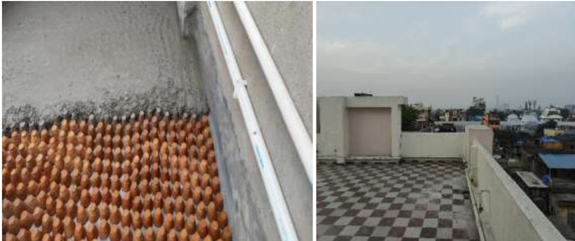
Water proofing and heat insulating treatment over roof
