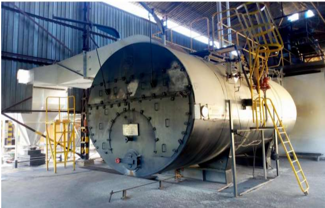
Fig1. Firetube boiler
