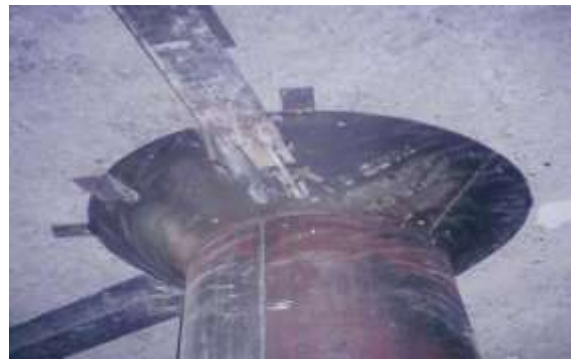
Figure 5. Steel plate bonding
