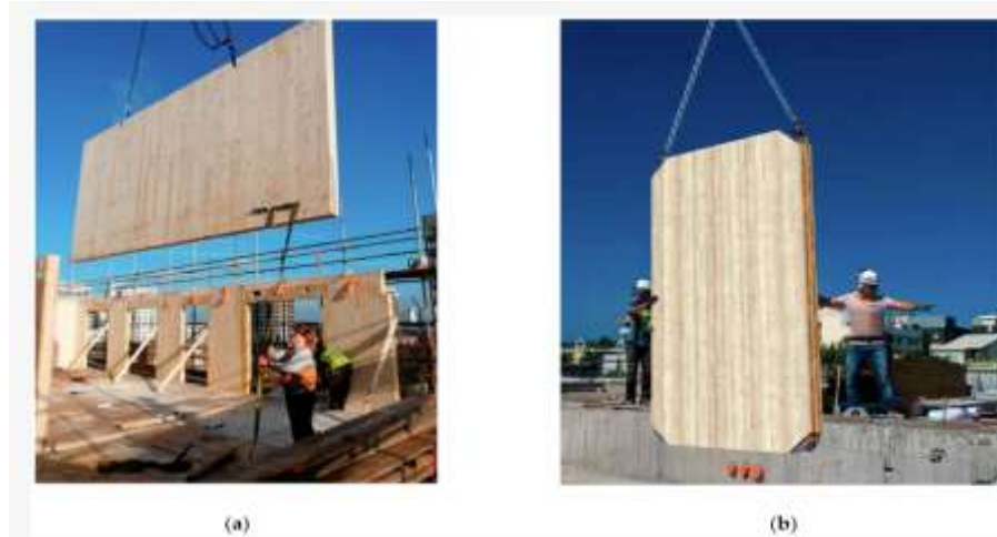
Figure . Panel lifting with (a) the conventional method and (b) novel connectors (CLT-C2)
