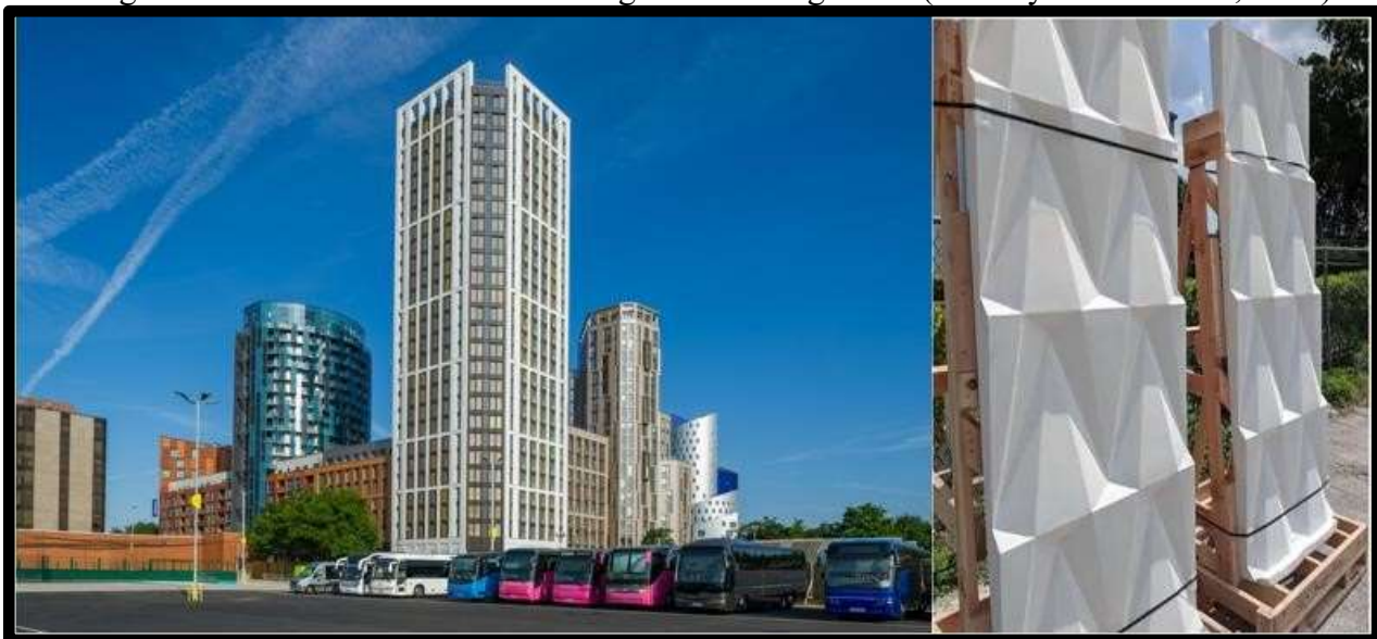
Figure 4.1: The Apex House project in Wembley and its employment of precast panels
