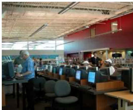
Fig.1 ‘Semiahmoo Library, Surrey, B.C.: The project uses a very simple exposed structure consisting of W sections and OWSJ with a painted finish’ (Boake, B.E.S., B.Arch., M.Arch., & AP, 2012).
