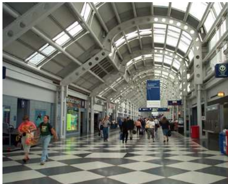
Fig.4 ‘O’Hare International Airport in Chicago was the first airport to use AESS. The complex nature of the sections and connections called for a tighter sizing tolerance and even finish application’ (Boake, B.E.S., B.Arch., M.Arch., & AP, 2012).
