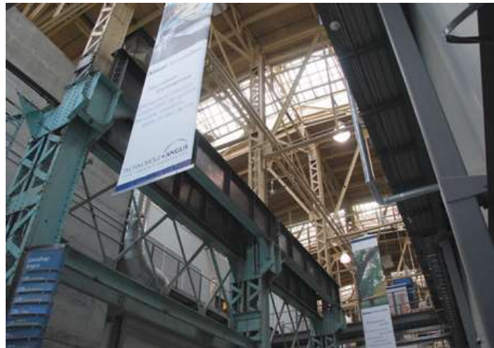
‘Fig.8 Angus Technopole, Montreal is a unique reuse application of a former locomotive shop as offices and commercial space. New steel is required in this project, a custom specification is required in order to make it fit into the aesthetics of the old building’ (Boake, B.E.S., B.Arch., M.Arch., & AP, 2012).
