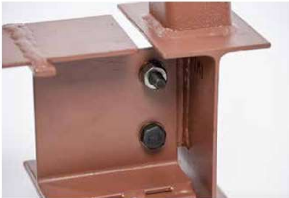
▲ SSS: Bolt head orientation not defined.
