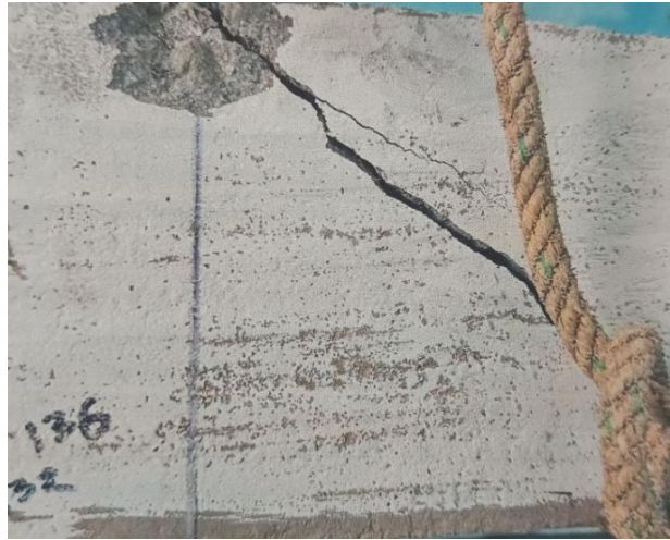
Figure 10: Failure pattern of crack at shear zone
