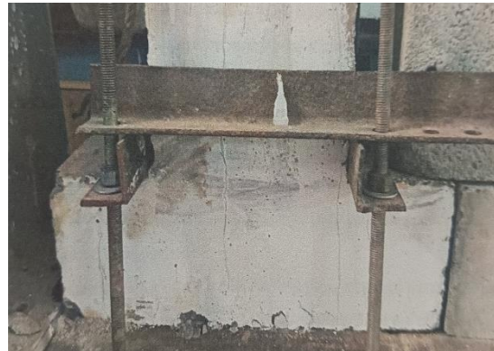
Figure 7: Crushing of column at end
