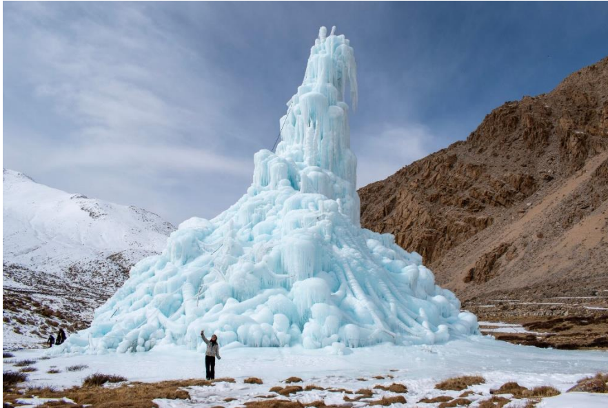
Figure 1 . Ice Stupa used for water conservation in Ladakh. Source: Lyons, Kleinman Center for Energy Policy Website.
