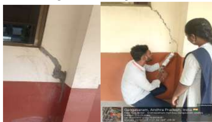
Figure 5: Crack repair works
