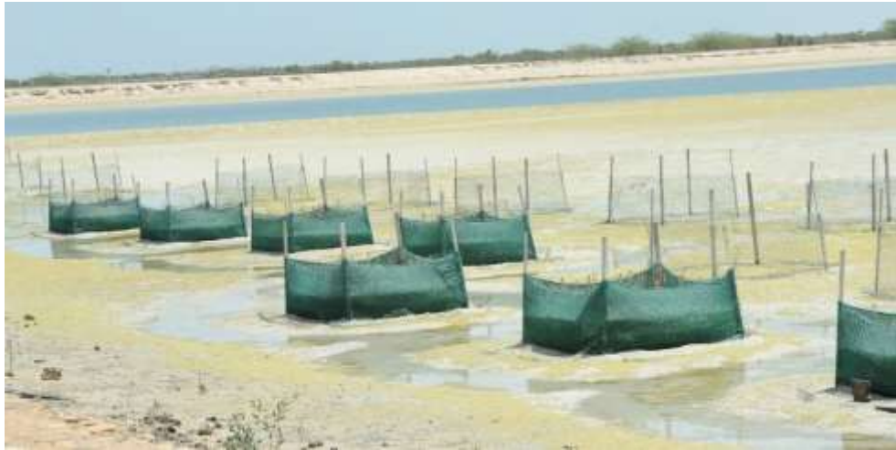
Figure (2): Showing Completed Dispersal Centers formation and stabilization using mesh fencing
