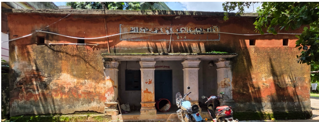
Figure: No-6- Police station, Anandapur
