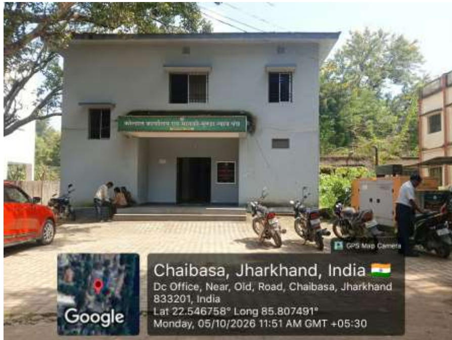
Source:- Image taken during field visit. New building of the Manki Munda Court, SDO office campus, Chaibasa, West Singhnhum, Jharkhand, near Civil Court , Chaibasa
