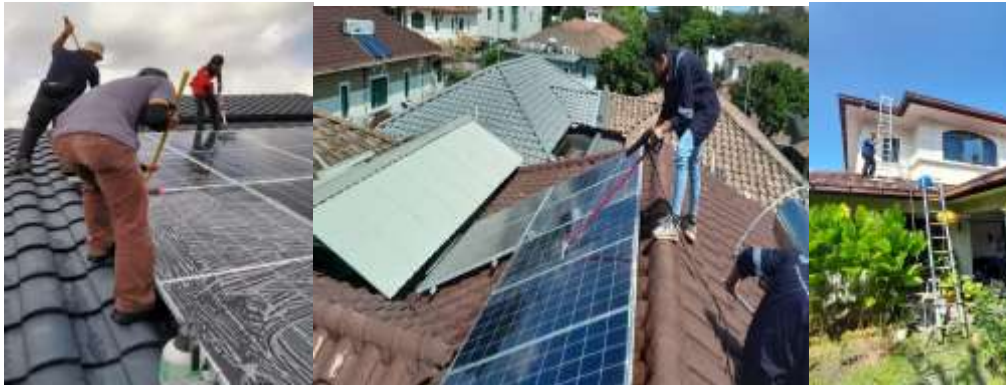
Figure 2: Conventional manual rooftop solar PV cleaning at height during maintenance operations.
