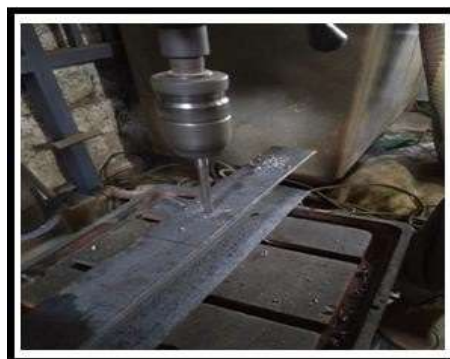
Fig.5.4.1 Drilling of C-Channel
