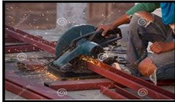
Fig.5.5.1CuttingofC-Chanel
